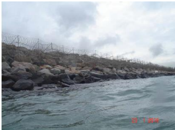
Artificial Sloping Seawall with Boulders
